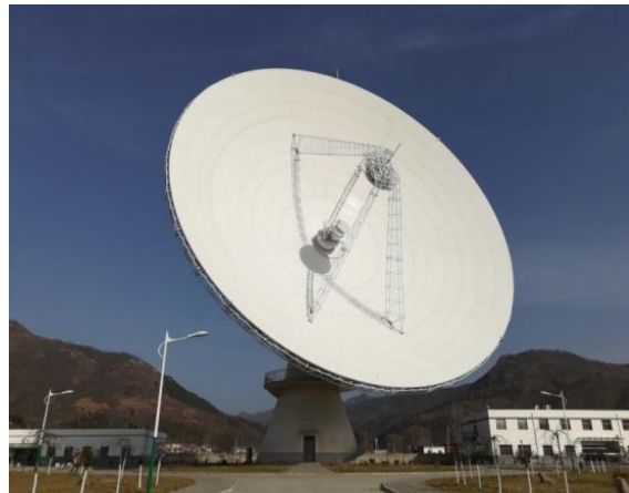
Fig.1 40-meters parabolic antenna appearance
